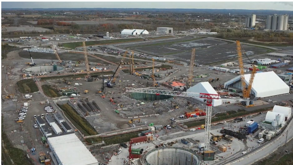
Figure 7: Construction site of BWRX-300, Darlington site in Ontario. Photo credits GE Vernova
