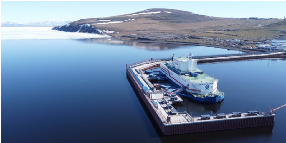
Figure 6: SMR Akademik Lomonosov, the floating power unit (FPU), based in Pevek, Chukotka (Russia's Far East), photo credits Rosatom.
