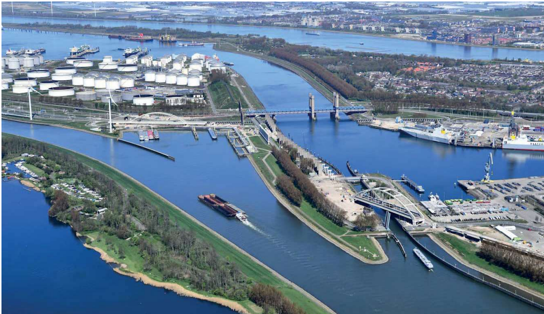
■ There are more than 40 industrial sites across the port of Rotterdam, all with different energy needs
